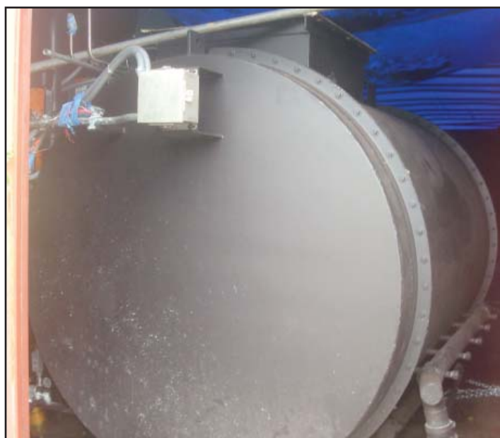
The new incinerator has been sitting as the incineration site for months, waiting to be installed.
