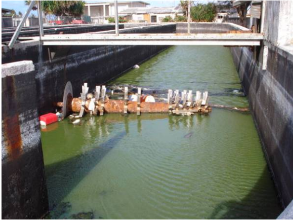
Non-operational sewer treatment plant
