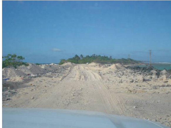
Portion of the unprotected causeway
