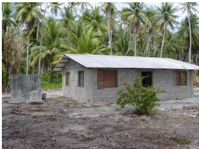
Health Center: Under construction (Plans underway for completion)
