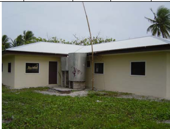
Health center: Rear elevation with steel water tank
