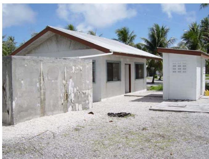
Health Center: Rear view
