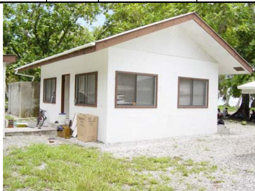
Health Center: Rear view
