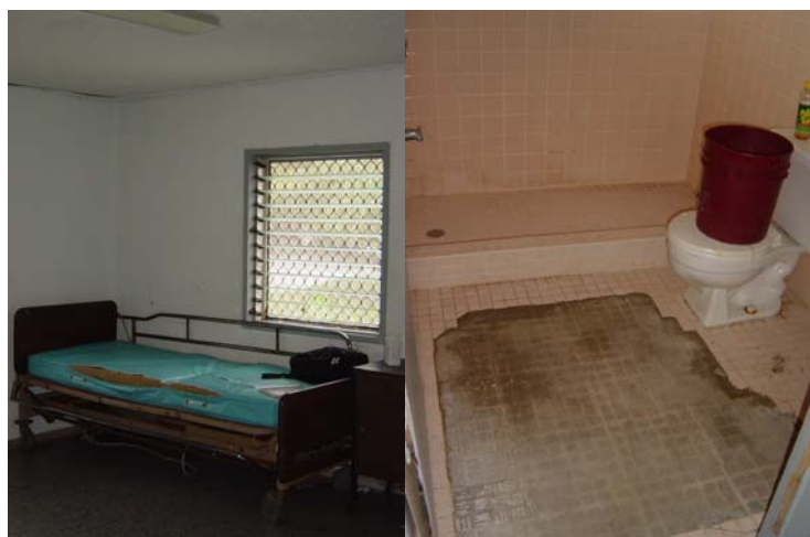
Health Center: Inpatient room and Toilet & shower
